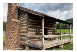
◀ B&C Masonry, did an amazing job on the Davis Cabin chimney and fireplace! Except for the firebrick inside, the fireplace and hearth were constructed using only the 200-year-old brick salvaged from the original structure. The masons mimicked the crudity of the original joint work!
