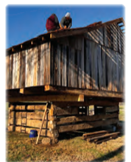
Freddie Haun and his reconstruction team work in November to install the roof atop the cantilever barn.
