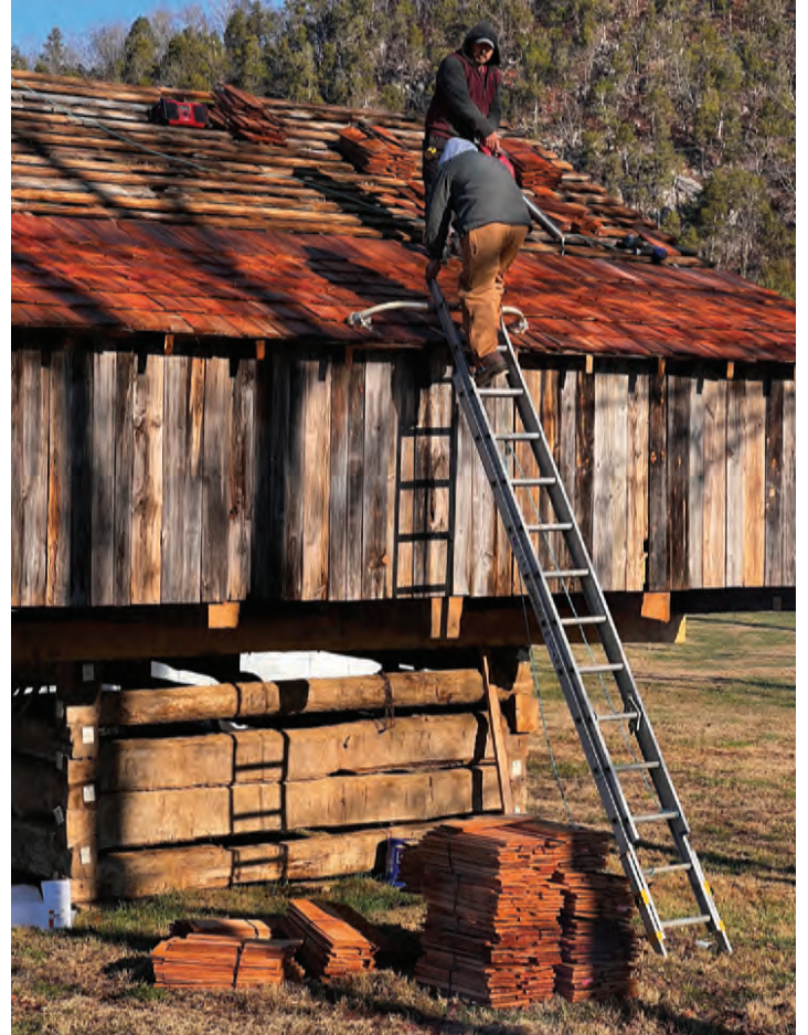
Freddie Haun and his reconstruction team work in November to install the roof atop the cantilever barn.
